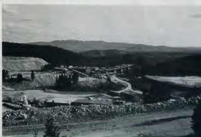
Nerco Minerals' DeLamar Mine closed vat cyanide leach plant. Owyhee County, Idaho.
