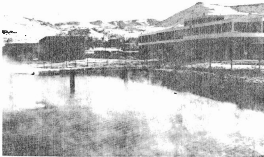
The cooling-pond used with the State of Idaho health-agriculture building in the background.
