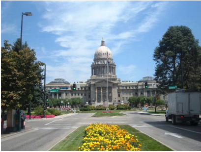
The geothermal-heated Idaho State Capitol. Photo taken by Daniel Fleischmann, GEA
