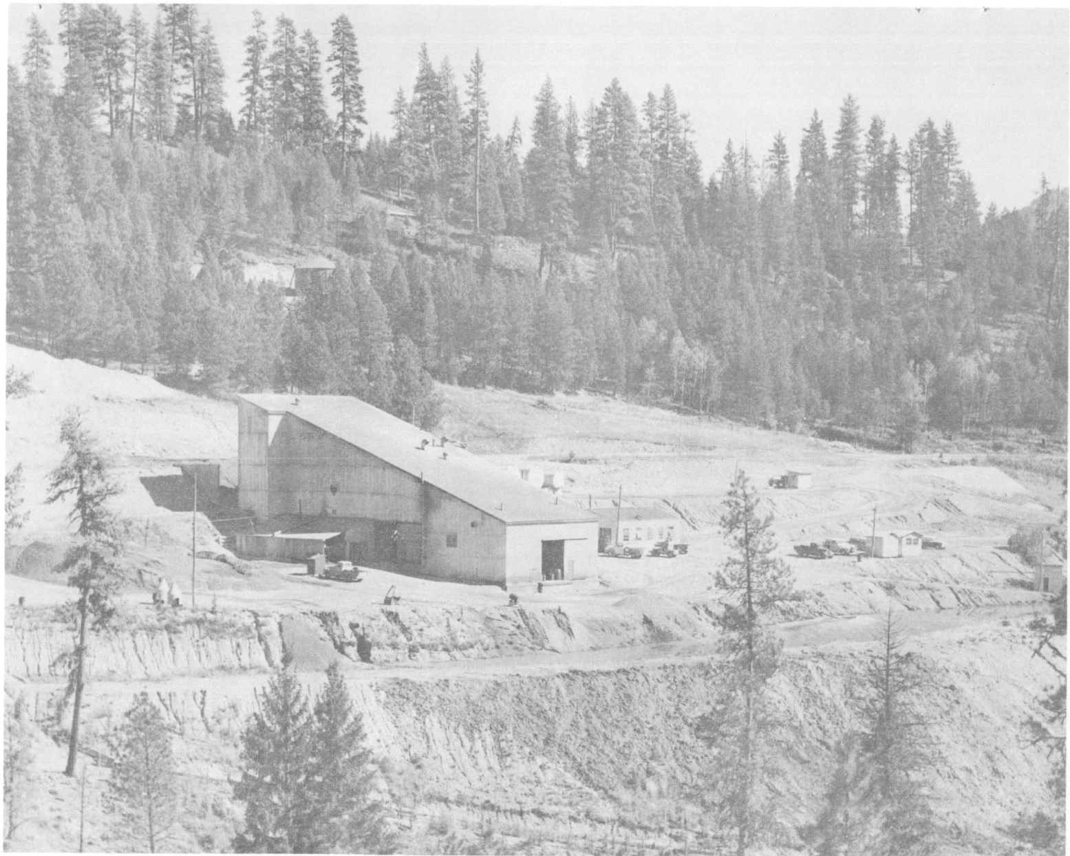
Figure 1. Blacksand separation plant designed to recover columbite, euxenite and monazite; ilmenite, magnetite, zircon, and garnet are by-products. Operated by Porter Bros. Corporation at Lowman, Idaho. Treatment of dredge concentrates at this mill includes: electromagnetic, high tension electrostatic, and gravity separation. Capacity of the mill is 150 to 200 tons per day; recovery is 88.44 percent.
