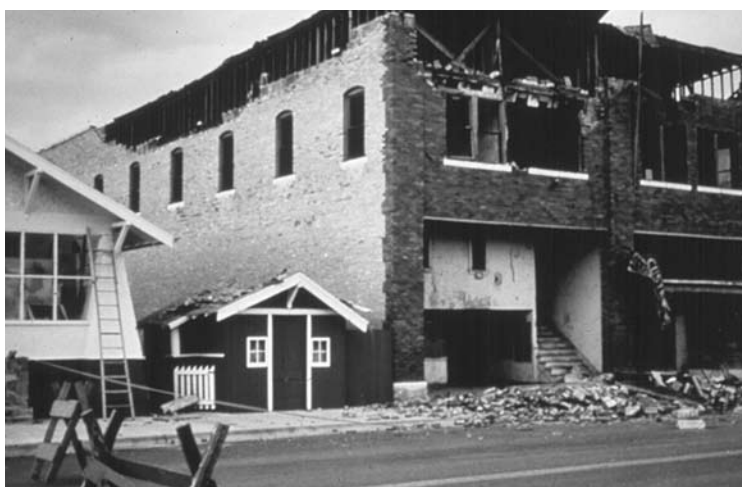
Earthquake damage to Custer Hotel in Mackay.
