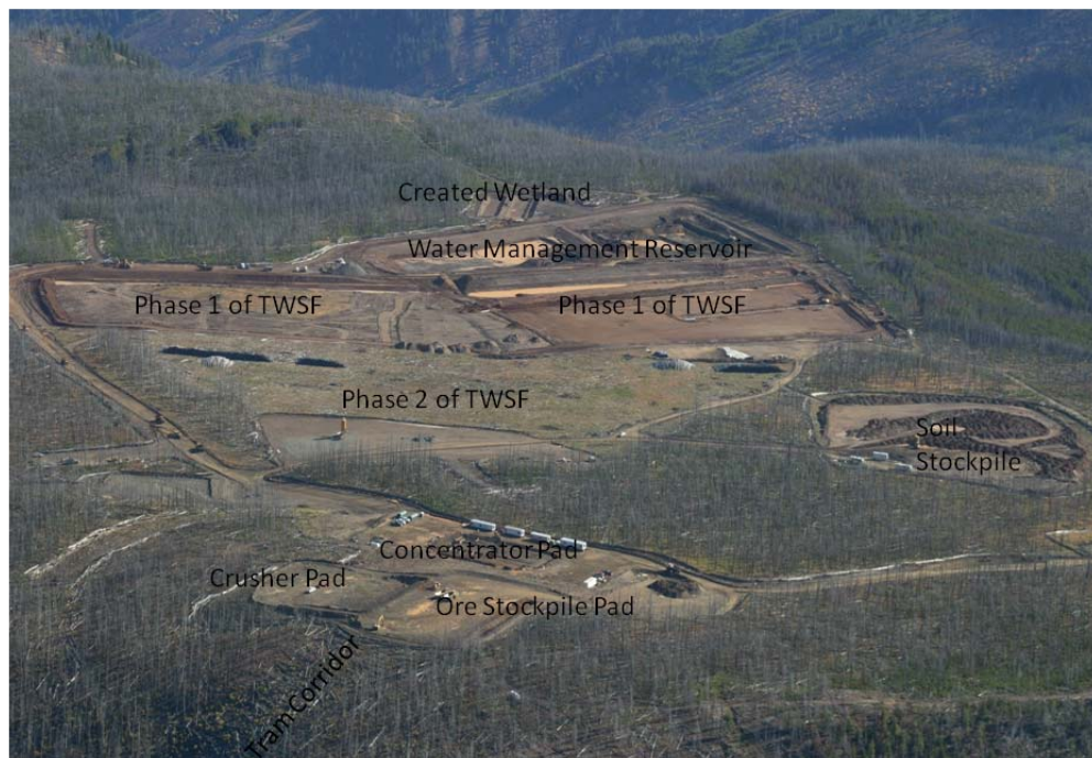
Figure 15. Idaho Cobalt Project under construction by Formation Metals, Lemhi County.
