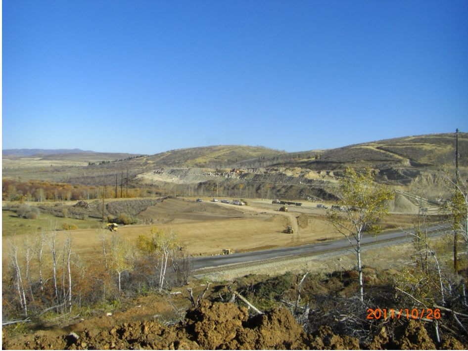
Figure 7. Construction work at Monsanto's new Blackfoot Bridge phosphate mine.
